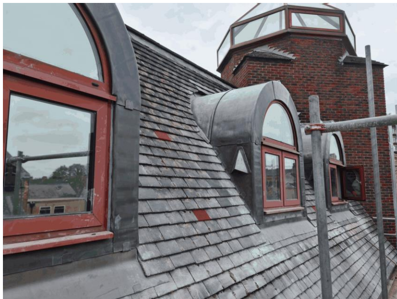
(new church roof)
